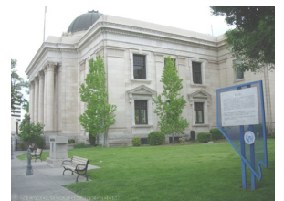
Virginia Street at the Washoe County Courthouse -- Reno
