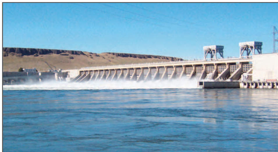
As an engineer in the late '40s, Ethel Birnbach worked on designing McNary Dam near Hermiston, Ore.
