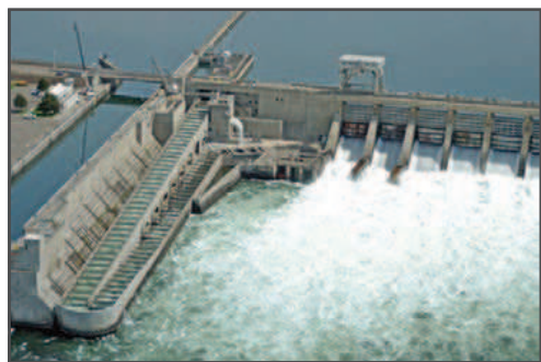
The fish ladder at McNary Dam, designed by Ethel Bimbach and the Army Corps of Engineers, is at left.
